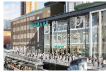
FORUM Rotterdam, Rotterdam (under construction)
